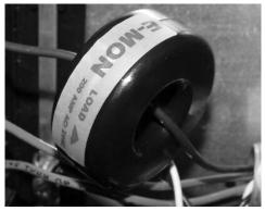
Fig. 5. Solid-core Current Sensor
